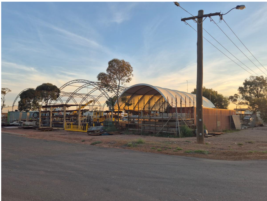
Figure 1: Two partially constructed dome structures located adjacent to a completed dome structure on a corner lot.
