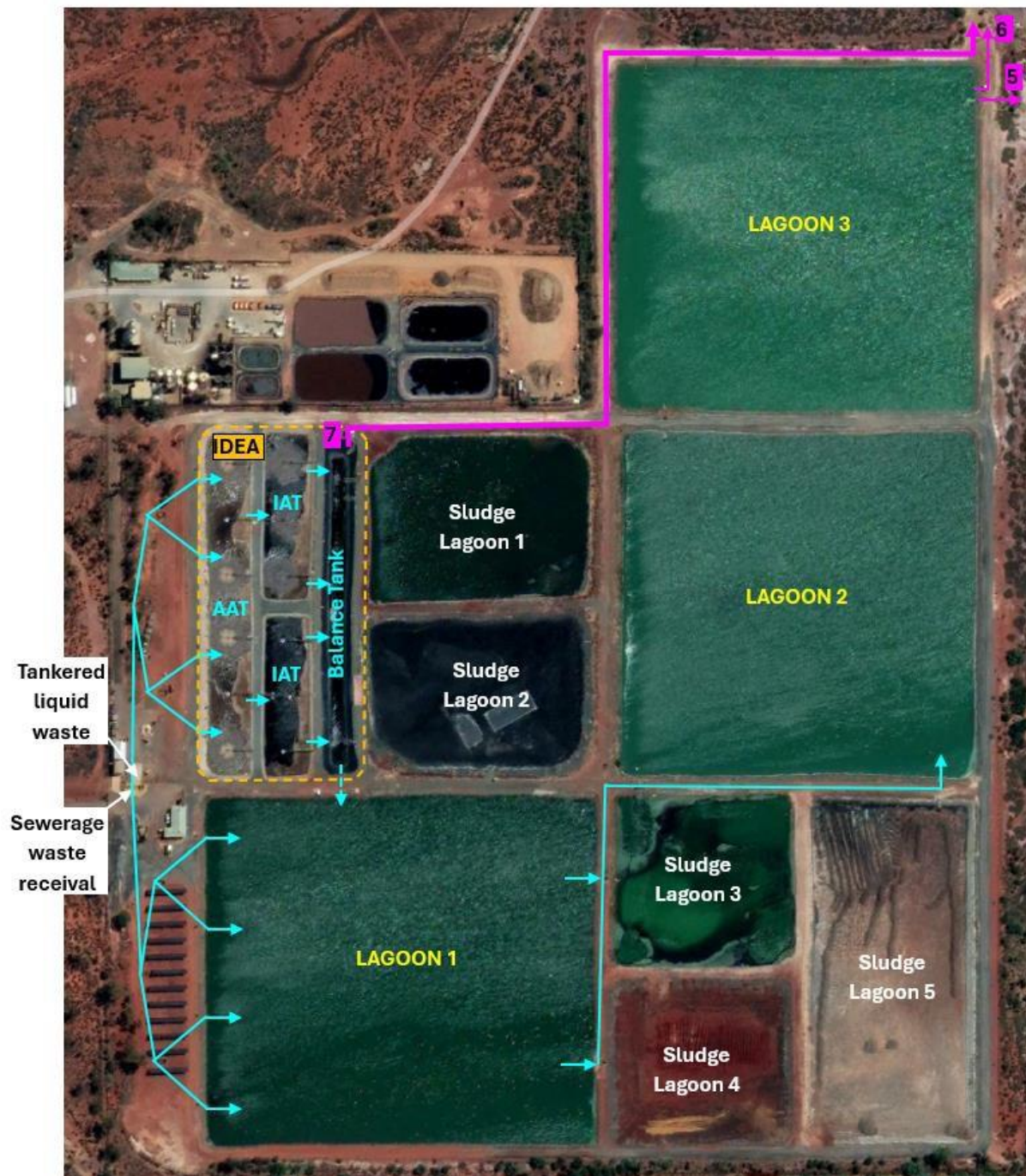
Figure 3: SBWWTP prior to 2020
